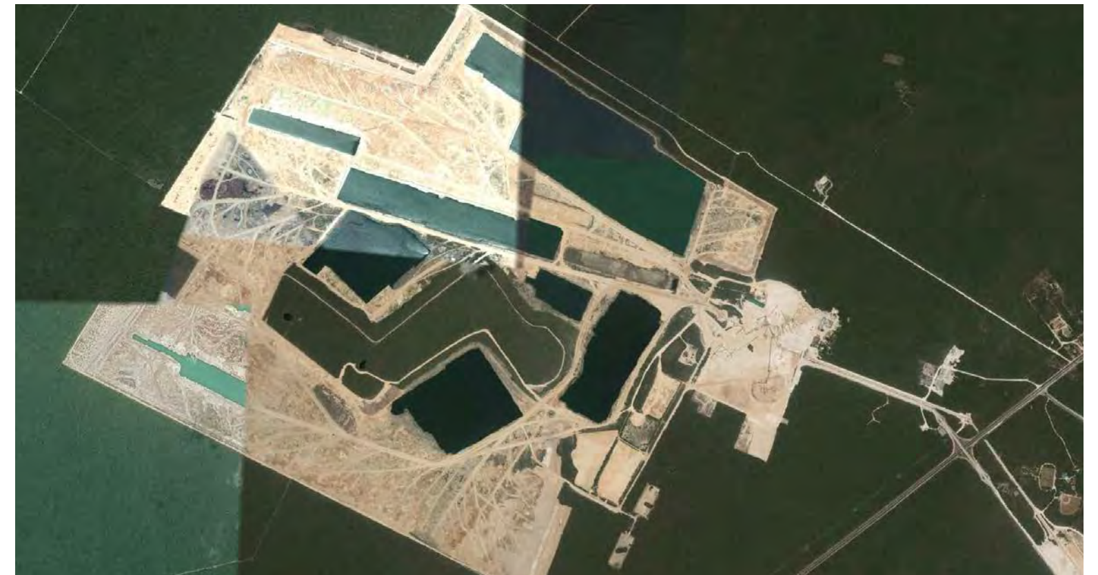
Water reclamation and collection plant outside Playa Del Carmen
