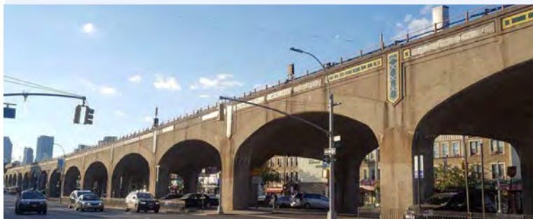
OVERHEAD TRAIN STRUCTURE
