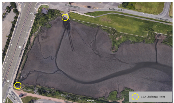
Aerial of CSO outfall locations located within the site.
